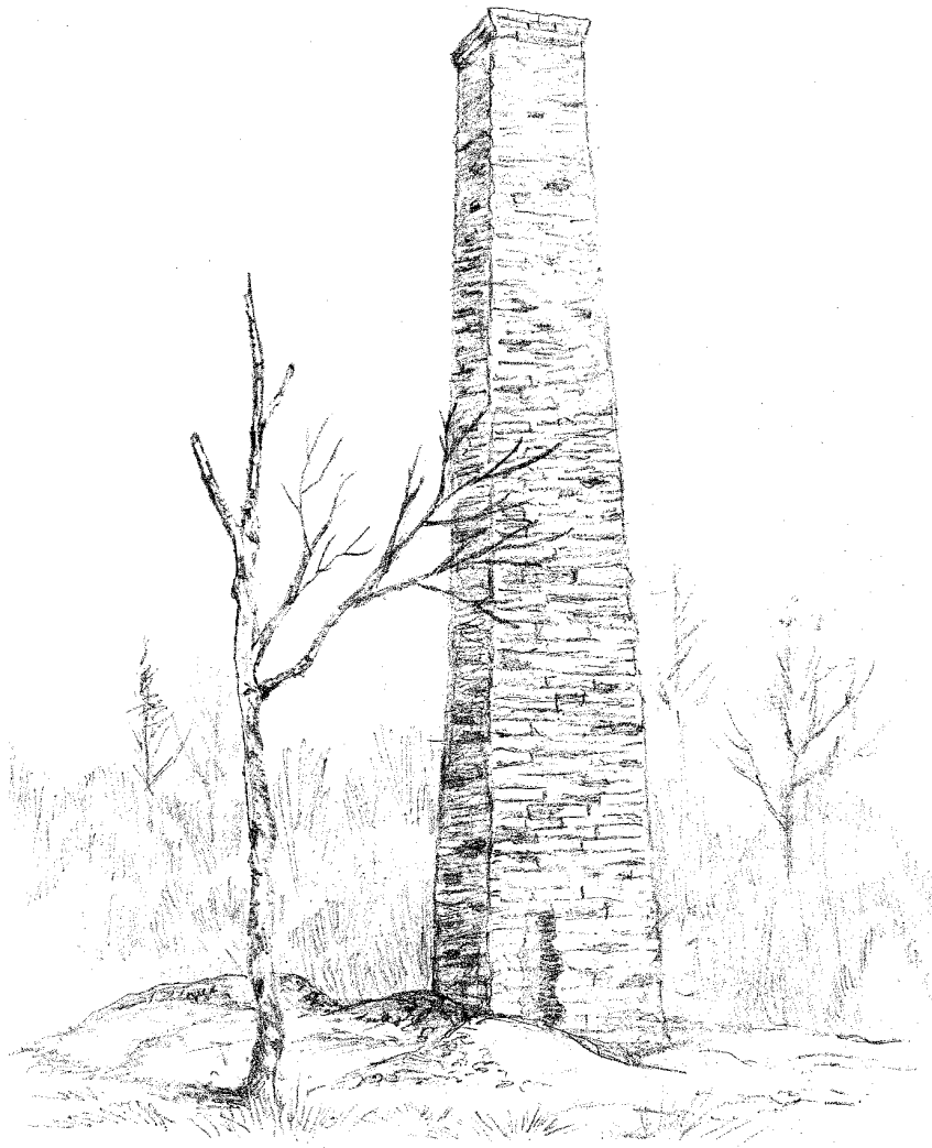
Chimney at Victoria Vein, Rossie. SR
